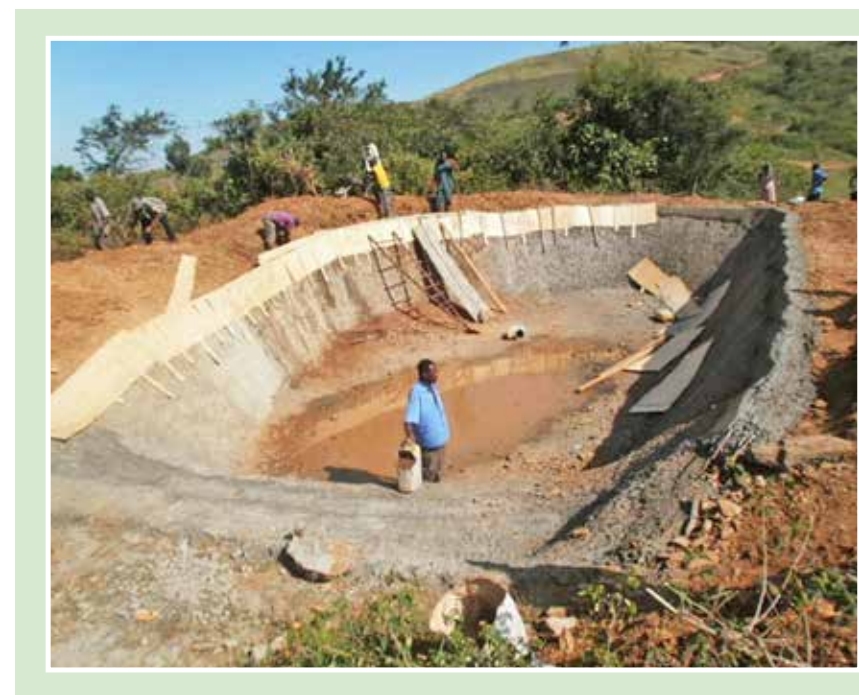
Members of Kashari community participating in the construction of their water reservoir, 2010
