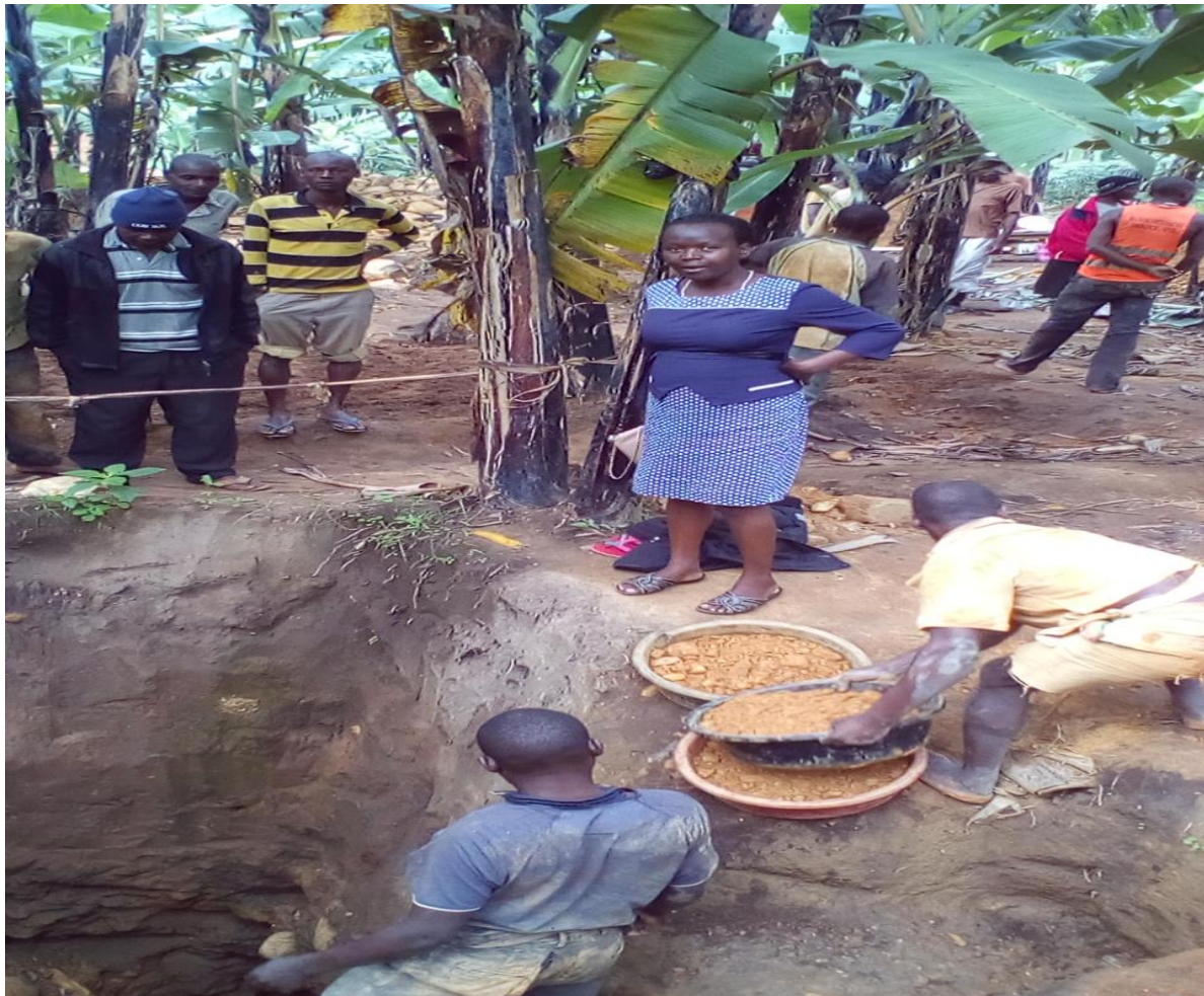
Photo 4: Low technology/inappropriate tools, no PPEs
