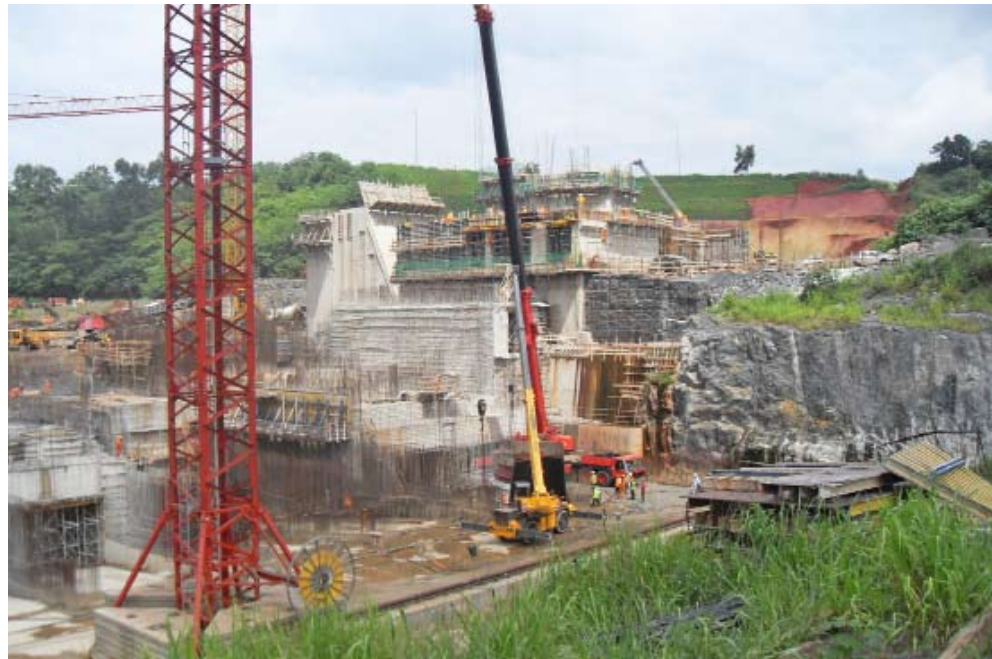
Unending problems with Bujagali dam: a new design in the offing!
