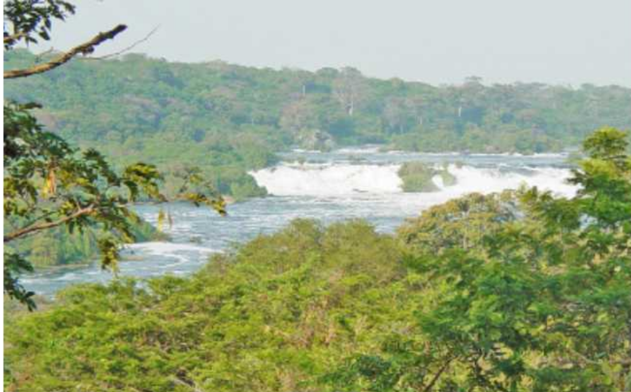
Karuma Falls on River Nile where the Karuma dam will be constructed
