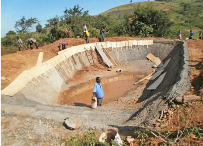
NAPE working with a community in Kashari to construct a water reservoir, 2011
