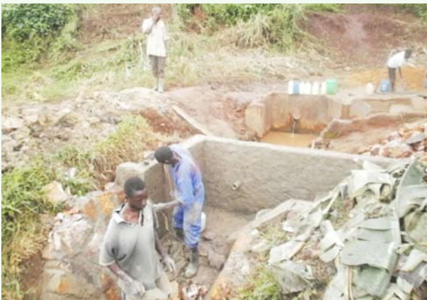
A community in Mukono rehabilitating a protected well with support from NAPE
