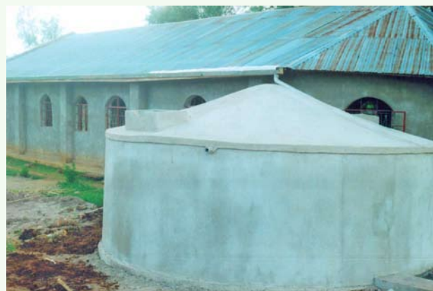
NAPE constructed a rain water harvesting tank (300,000m 3 ) for a water stressed community in Luwero
