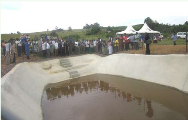
NAPE constructed a water reservoir (700,000m 3 ) for a water stressed community in Kashari, Mbarara
