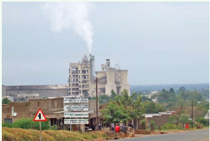
Hima Cement factory, Kasese, Western Uganda
