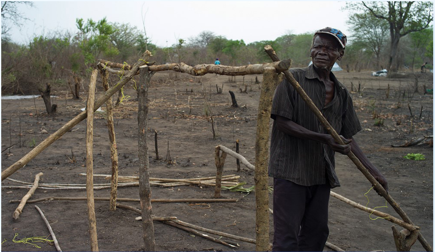
A refugee building a makeshift for his family in Palorinya Refugee Settlement, Moyo District. Photo credit: Dan Kitwood
