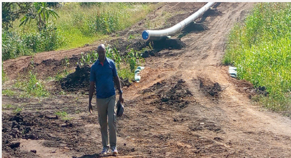
East African crude Oil Pipeline EACOP snaking through Nyakabingo village, kabaale parish, Buseruka Sub county –Hoima District as of June 13th 2025.-NAPE file Photo.
