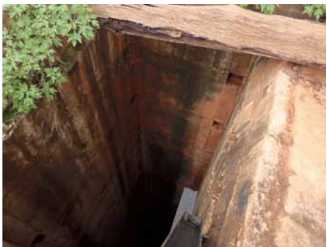
Good Practice: This tunnel in Geita – Tanzania was constructed during the colonial era with concrete; it has been in place for more than 50
