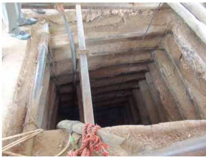
This tunnel in Geita – Tanzania is currently used by the Nsangano Gold mine Project; the embankments of the tunnels walls are made from wood planks.
