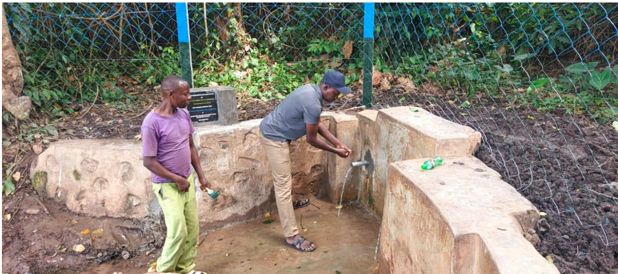
Plate 2. the repaired water spring back to normal water flow as was before blockage
